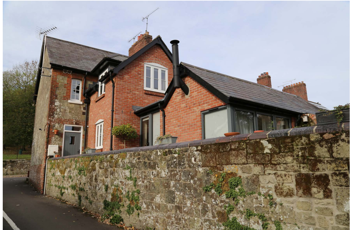
Contemporary extension to existing property St James's Street
