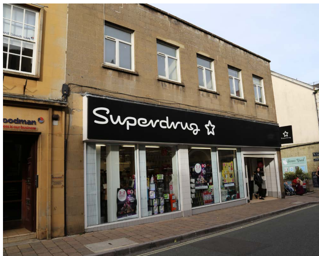
Poor quality shopfront High Street
