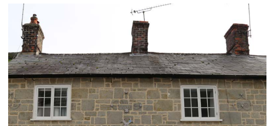
Chimney detailing found in Shaftesbury
