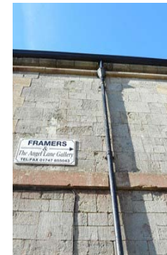
Classic half round gutter with round downpipes and traditional brackets in cast iron effect finish; hoppers can be varied but should allow for high capacity drainage
