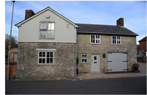
Contemporary renovation Haines Lane
