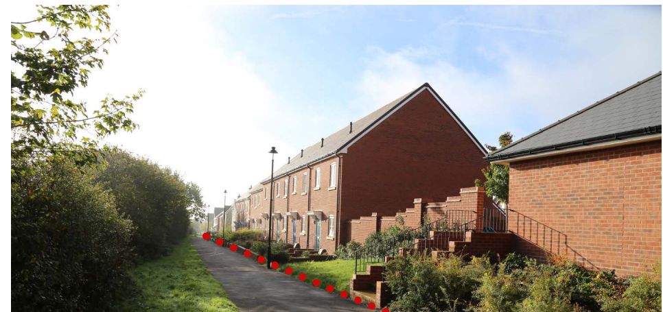
Above is a positive example, the red line delineates development edge fronting the green infrastructure corridor on Maple Road.
