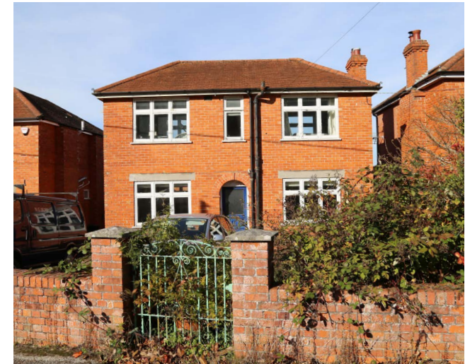
Post war property, Breach Lane
