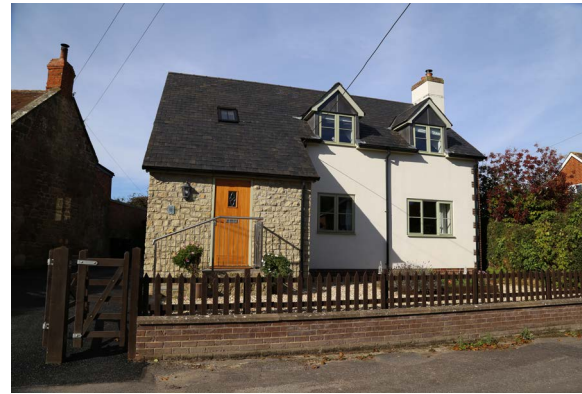
Contemporary renovation Well Lane
