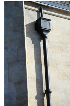
Classic half round gutter with round downpipes and traditional brackets in cast iron effect finish; hoppers can be varied but should allow for high capacity drainage
