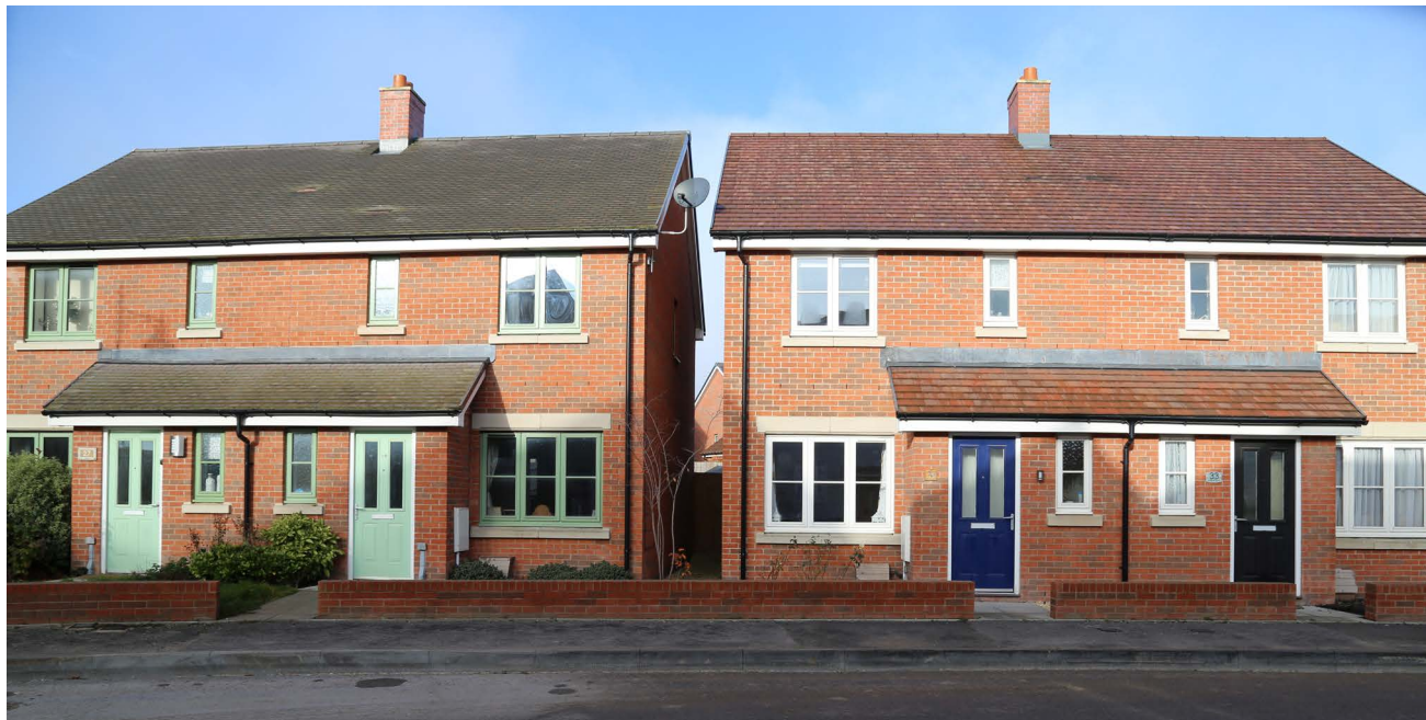
Recent housing development Maple Road. This development has attempted to reference the local vernacular, however there are issues with scale and density.
