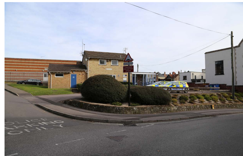
20th Century Police Station building
