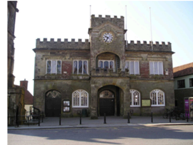
Town Hall internal renovations
