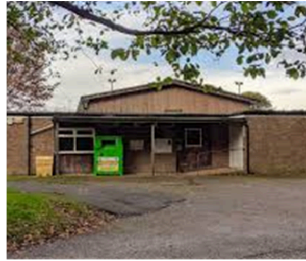
Youth Club renovation
