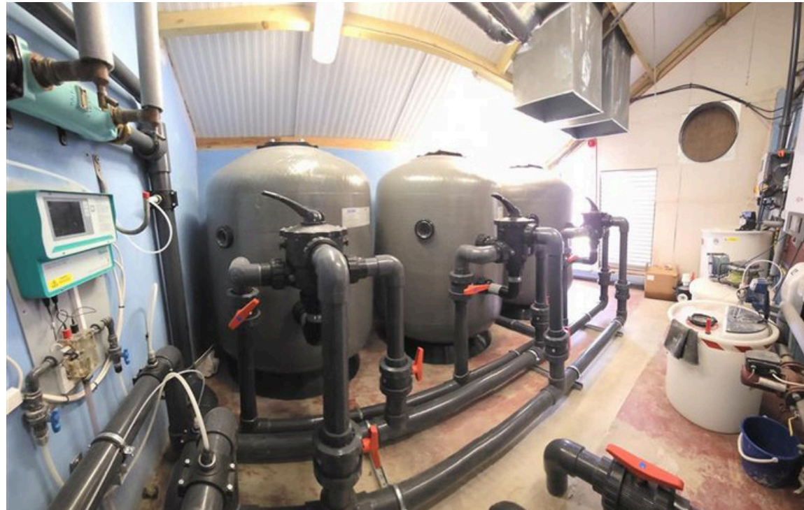
Lido new filtration system and pool liner
