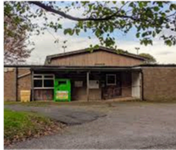
Youth Club renovation
