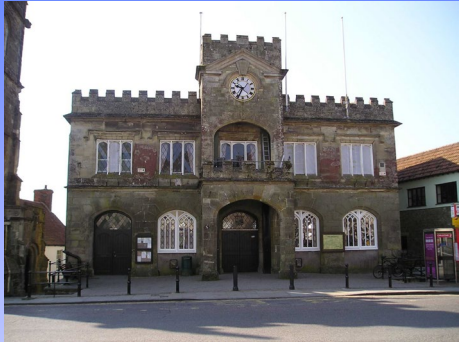
Town Hall Refurbishment £ 270,000
