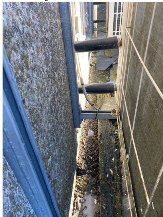
6: Gutter behind clock tower
