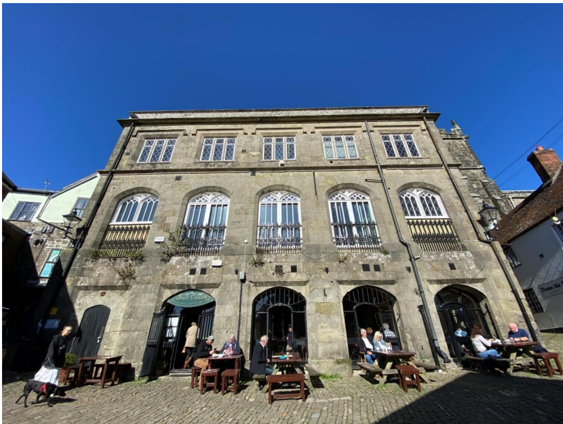
17. General view of South elevation. Plant growth, ties, vents and services.
