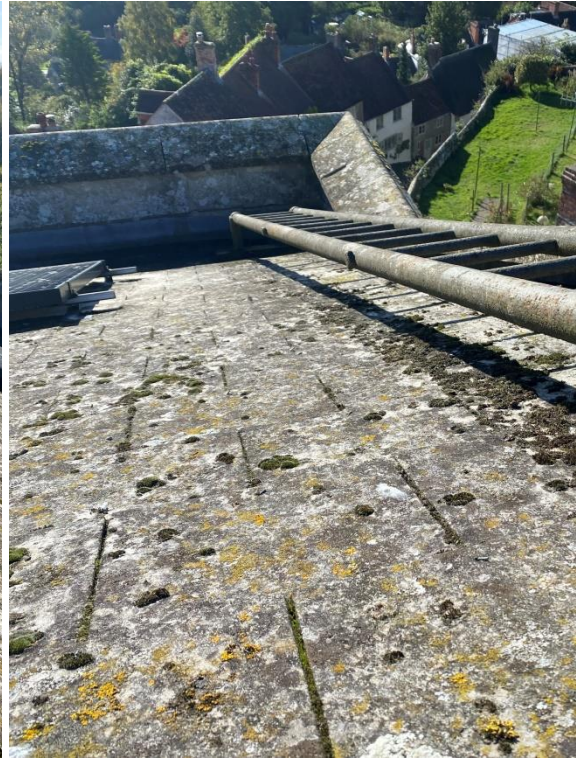
1: South roof slope, Asbestos slates, ridge and PVs 2: Access ladder to south roof slope, loose flashing
