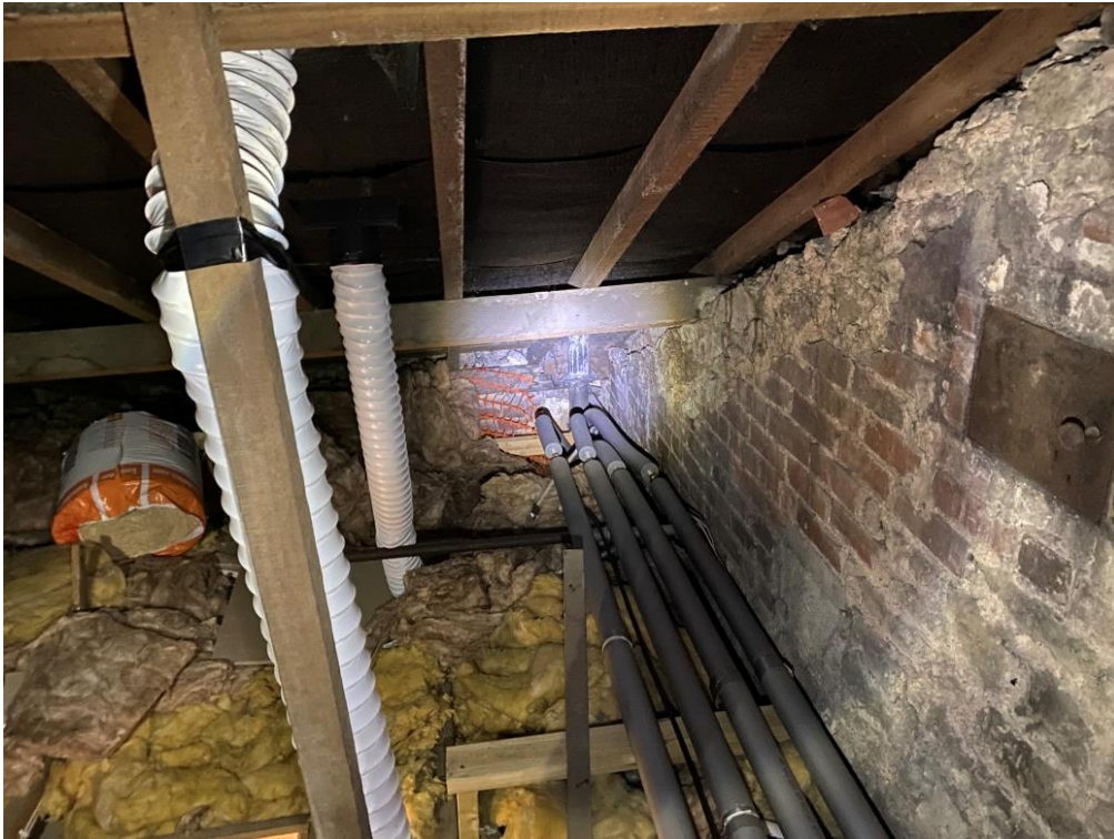
9: North East corner redundant lead soil stack, w.c. extract ducting, roll of unused insulation
