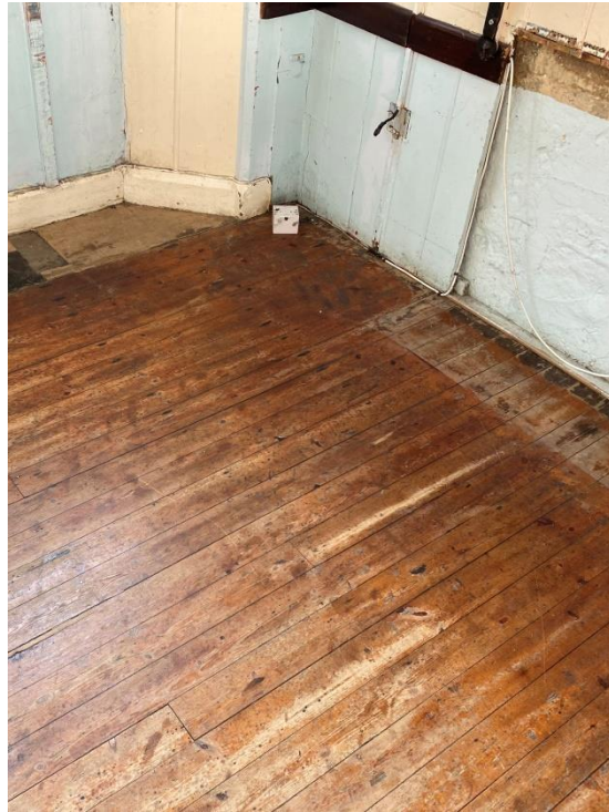
32: various floor finishes, patched walls, wiring SW
