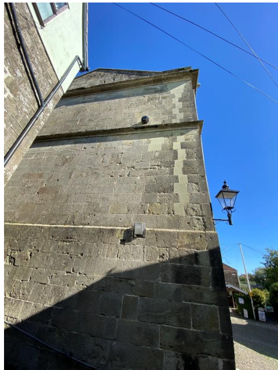
16: South West corner showing previous stone replacement
