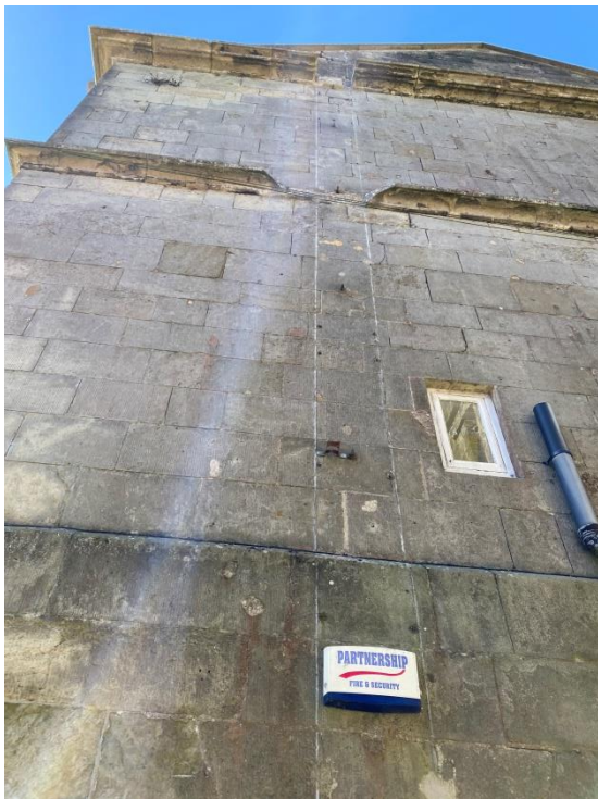
20: Scar from removal of flue
