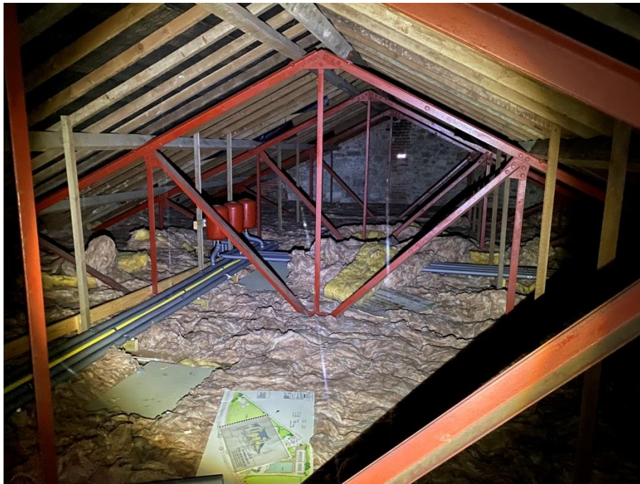
6: Roof space showing steel trusses, irregular untidy insulation, expansion vessels
