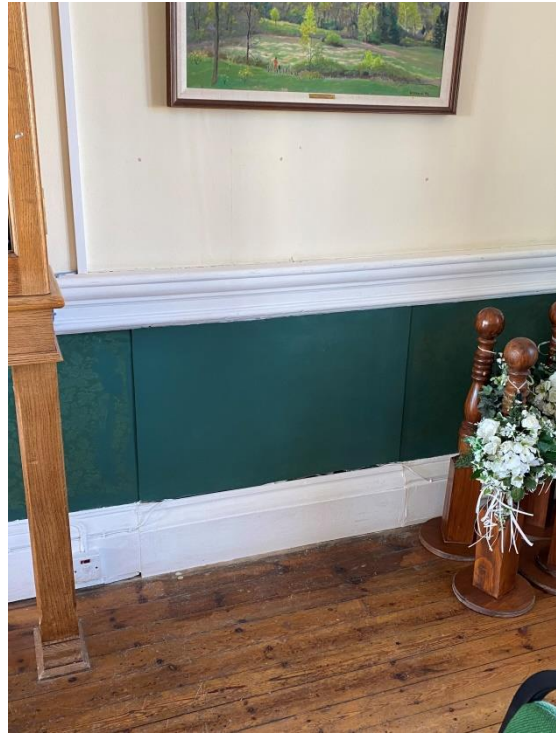
27: Patched wall where gas heater has been removed
