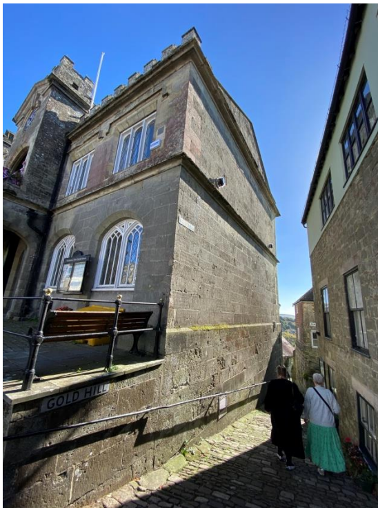
15: General view of West elevation
